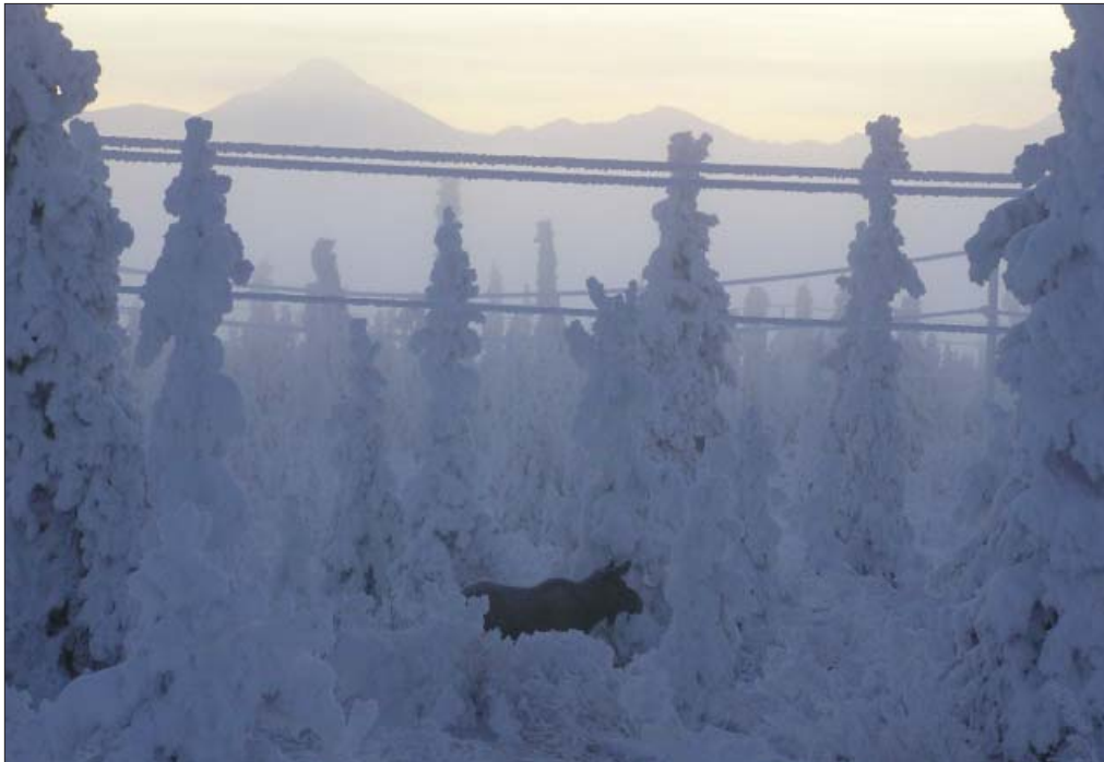
Lines near Eureka loaded with heavy snow and ice.
