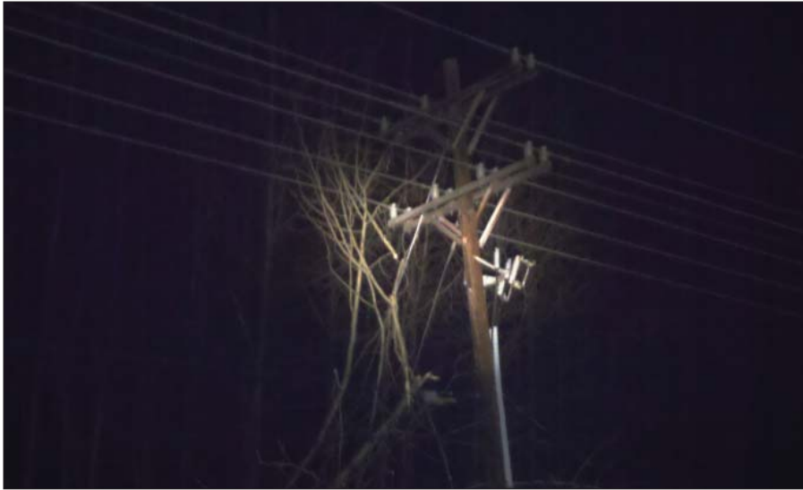
This tree on the power line in Valdez caused an outage for much of the community in November 2011.
