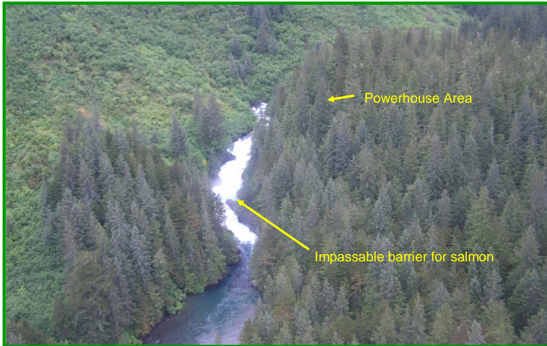
Figure 1.6 Silver Lake Powerhouse Location
