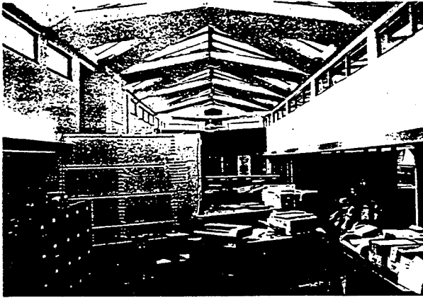
Conventional offices use half of their energy for lighting. Effective use of natural light, called "daylighting," dramatically reduces energy consumption at the time of day when the demand for electricity is the greatest. Photo: Donald Aitken.
